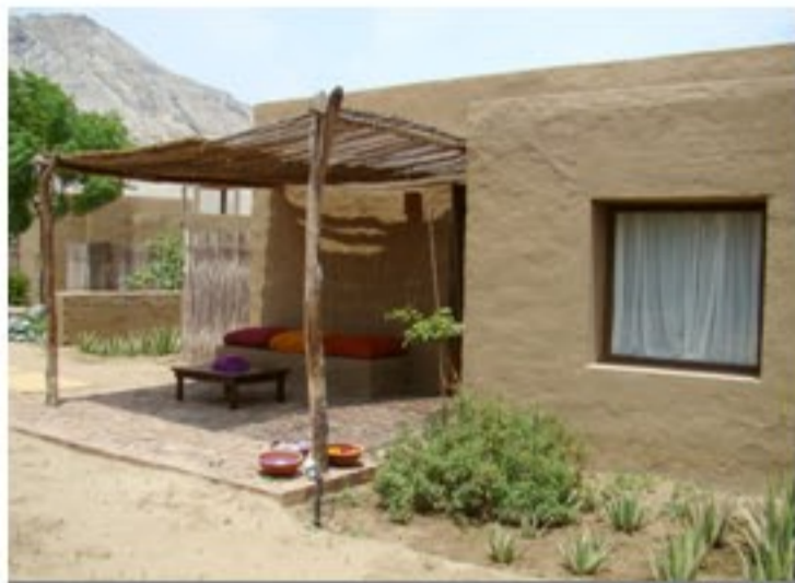
Boutique Hotel in Trujillo
